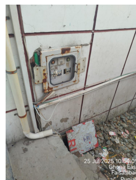
40. NC2. Broken electric panel.jpg
